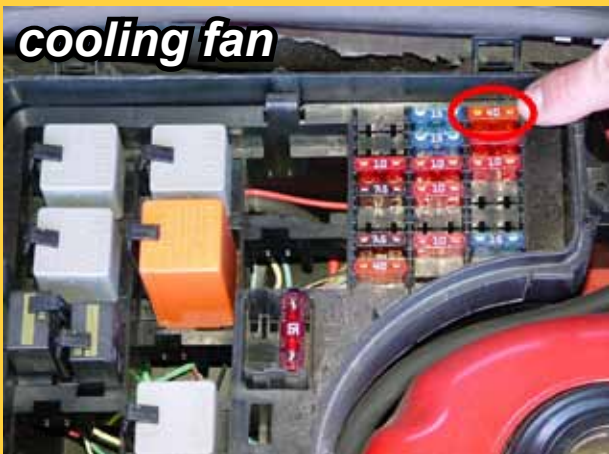
Remove fuse no. 3, located in the engine house.
